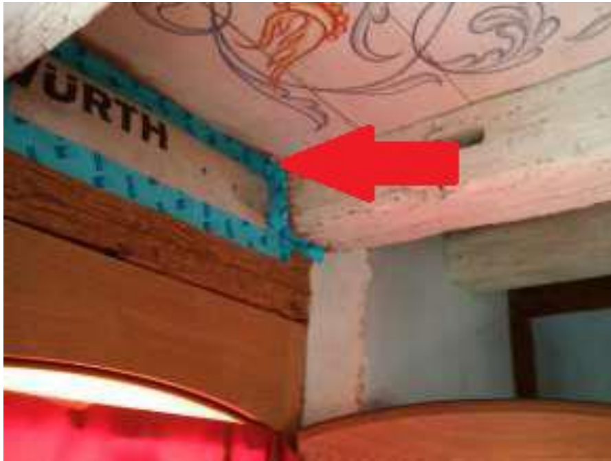
Special focus on wood beam end
