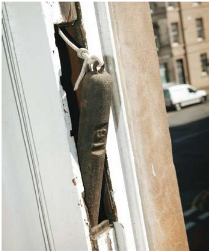
Sash weight exposed after removal of 'pocket piece'
