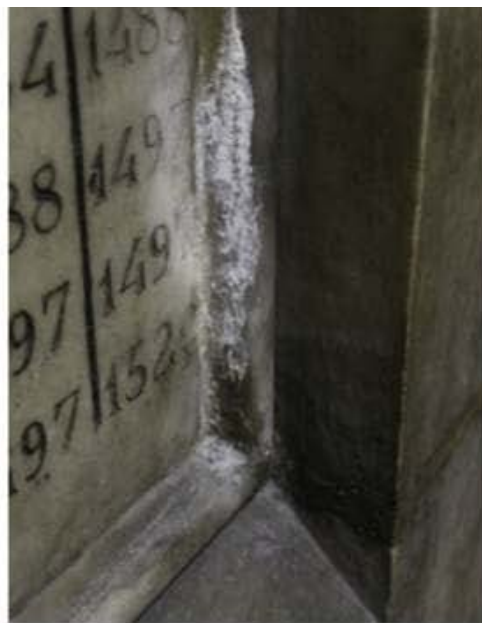
Efflorescence
